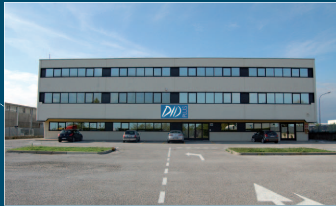
DID PLUS headquarters in Basiliano
